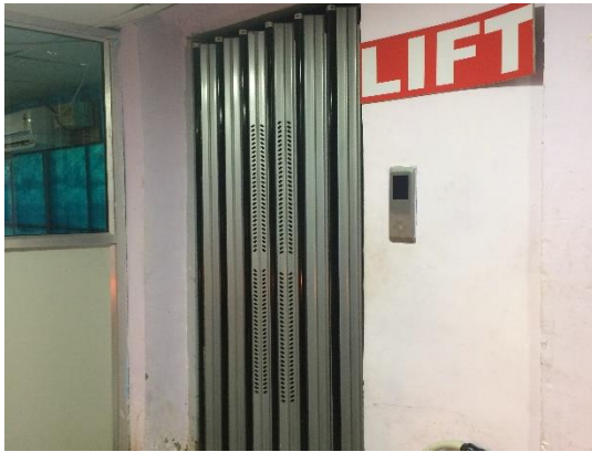
Lift Installation by Mr. Arjun Lamba sponsored by Help Age India.
